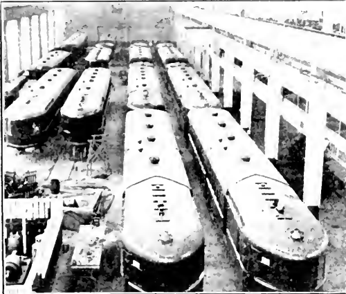
Petrol Electric Cars under Construction.
